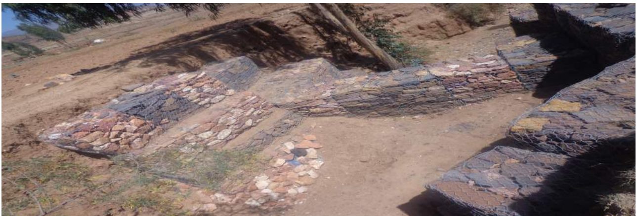
Picture xxxx Gabion Checkdam
